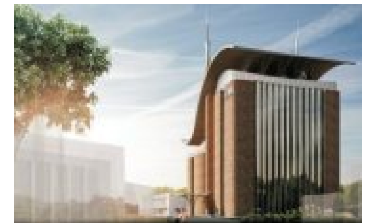
I&M Bank Head Office
